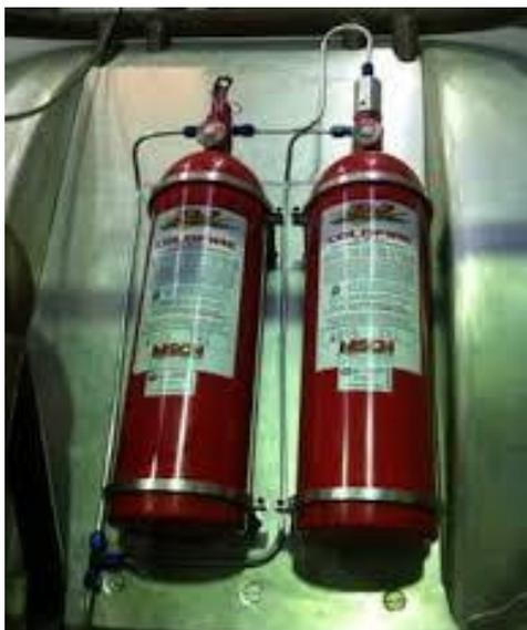
**NOTE:** It is a good idea to clean out the extinguisher lines and nozzles on a regular basis, using high pressure air (and some soapy water can help along with the air). Any queries with fire systems, please contact the Technical Chairman (See below).
